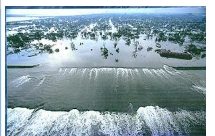
Image 4 – Levee breaking and flooding Orleans during Katrina
